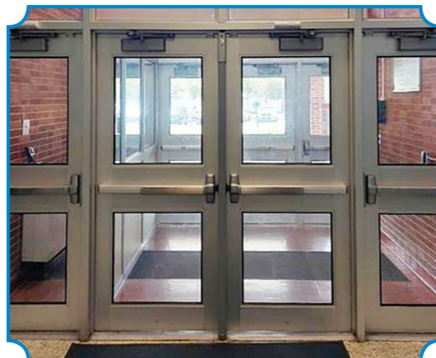
Each school has a double-door, single-person access control security space, also known as a mantrap, at the main entrance.
